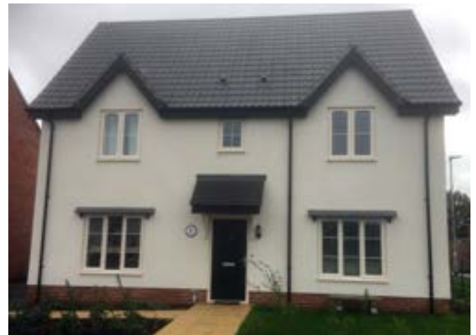
Rendered Ash GP blockwork
